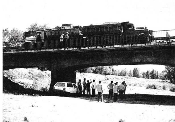
Figure 1 - Testing a bridge across the Vorskla river near the Bilyky village the Kobeliaky area after reconstruction
