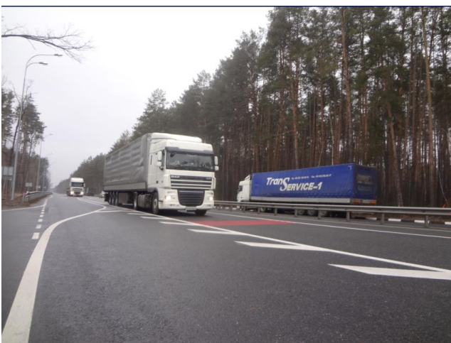
Figure 6 – General view of the ramp on PK 33+850
