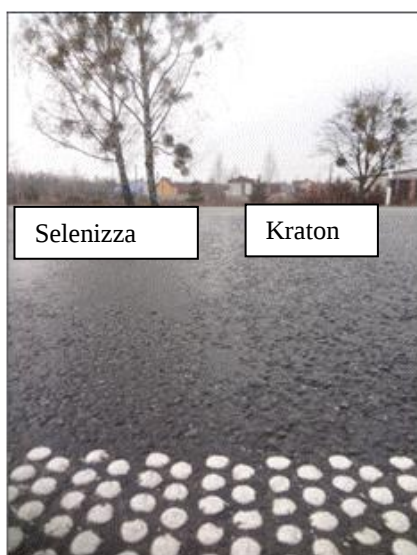
Figure 8 – Joint with SMA including Kraton (profile)
